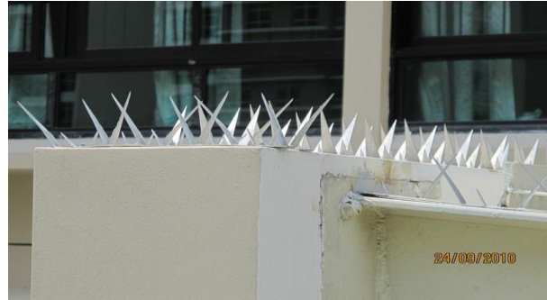
SPIKY20 – Perimeter / parapet Spikes Anti-climbing spikes on Perimeter or parapet. On Wall (Top) on Roof (below)
