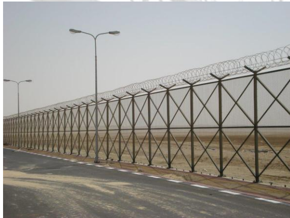
High Security Fence Installed somewhere deep in Middle East. GALFAN 95/5 + ORANGIC POWDER coating added life span.
