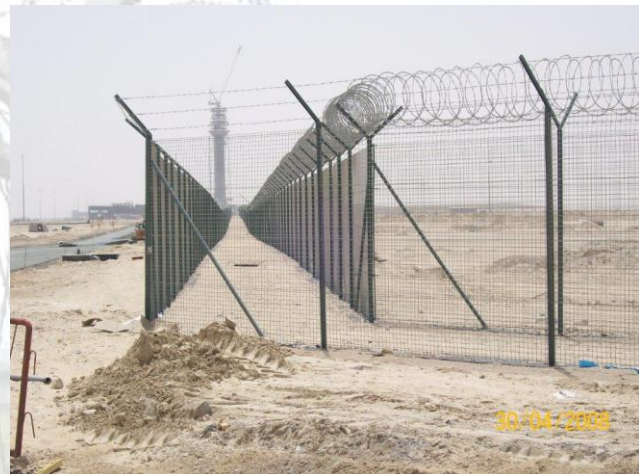
Double Mesh Fencing (GALFAN + Powder Coating).
